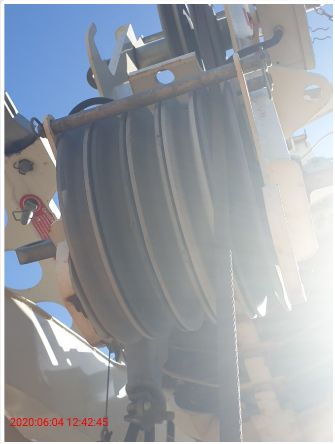
Head Sheaves and bearings
