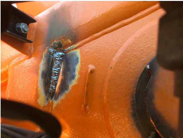
Photo 21: Repaired turret weld
