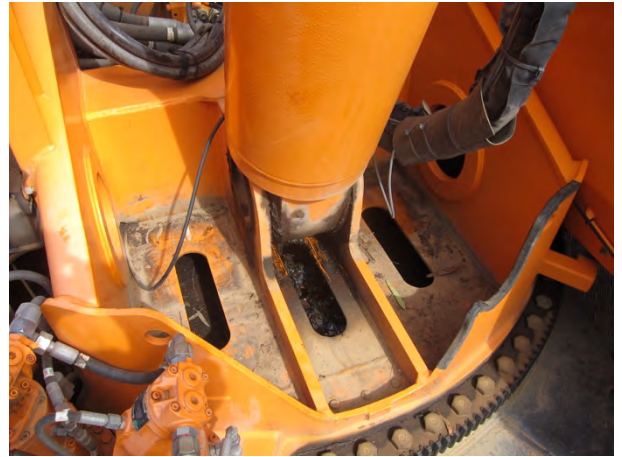
Photo 6: Lower luff cylinder weld and mount
