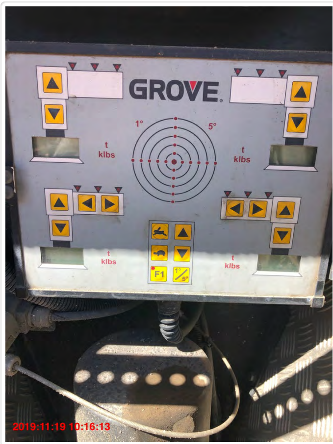
Outrigger Controls and Labeling
